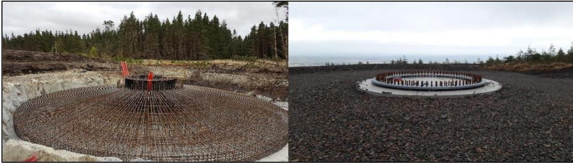
Plate 4-2 Turbine 'Anchor Cage' and finished turbine base
