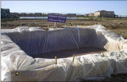
Plate 4-4 Concrete washout area
