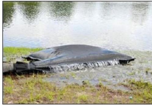
Plate 4-7 Silt bag under inspection
