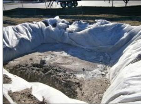
Plate 4-3 Concrete washout area
